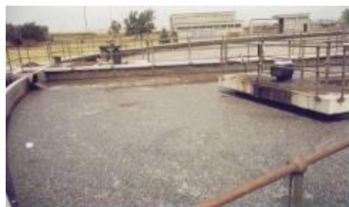
D. 2 weeks into dosing and the main solids have liquefied
