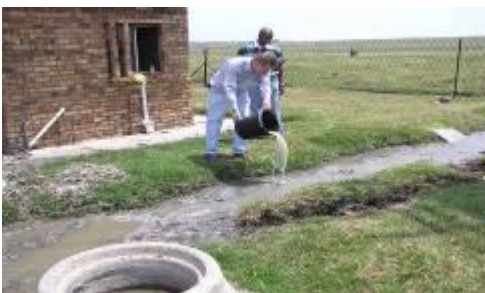
D. Dosing the product to biodegrade the effluent flowing to the river
