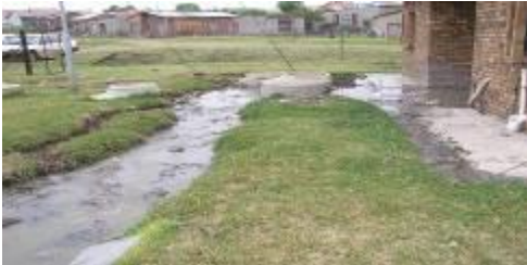
A. Raw sewerage running out of the pump station
